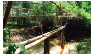
A traditional monkey bridge design constructed from bamboo
